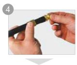
Immediately insert the expanded pipe end into the fitting until it reaches the last and largest ridge. Note the pipe contracts over time due to the PEX memory effect.
